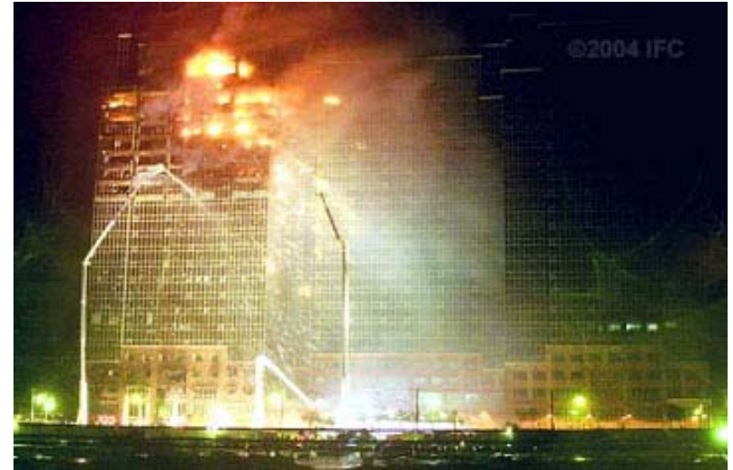
May 2001 - Taipei Office Building Fire started on 3rd Floor Spread and jumped to 26th Floor (Unauthorized removal of fire walls and lack of perimeter barrier firestopping hampered fire containment)
