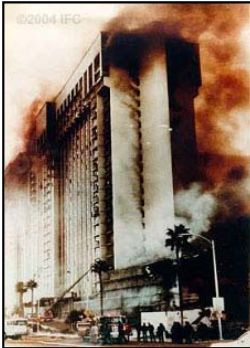
1980 MGM Grand Hotel 84 Died – 679 Injured Due to Smoke Propagation (Prior to Firestop Requirements)
