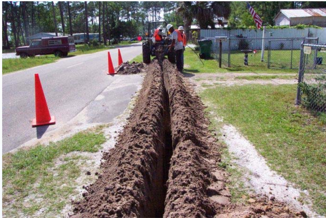
Trenching to place direct buried cable
