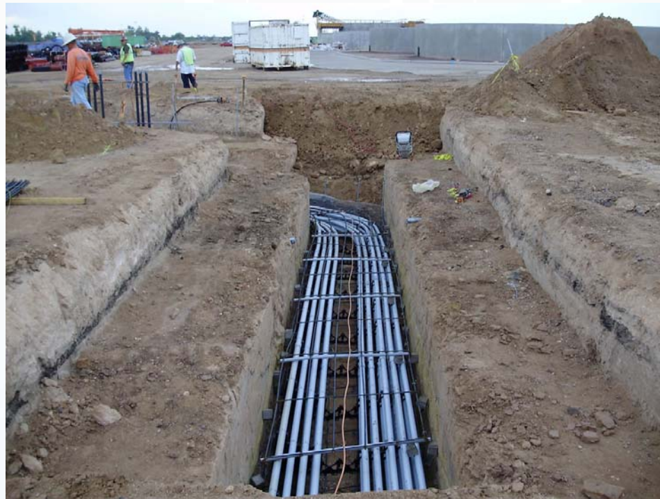
Underground Cable Placement
