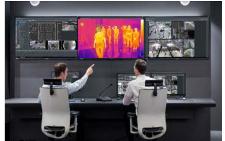
Manned monitoring station running Face Recognition & thermal analytical software
